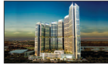
L&T Crescent Bay - Mumbai
