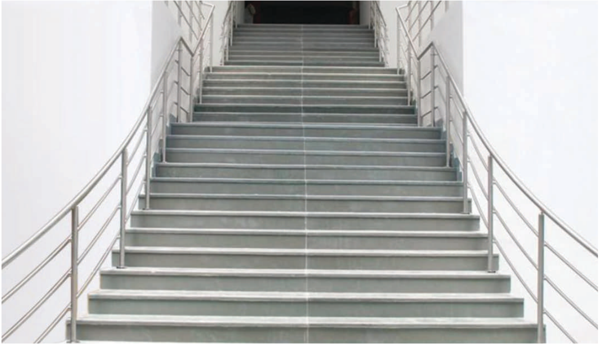
Top Mounted Round Baluster System With Horizontal Members - Ø 42.4mm (DT15-1-163) & Ø50mm(DT12-1-163)
